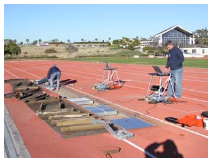
Force Platform Installation
