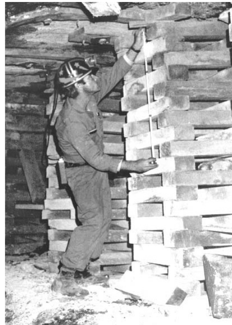
Measuring compression in support cribbing
